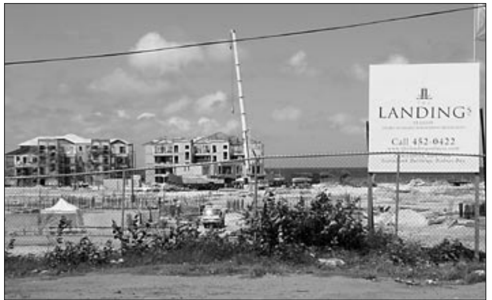
The Landings Construction Site
